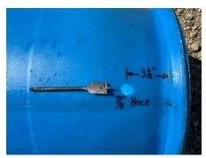
2. Three and a half inches up from the bottom of the barrel drill a 7/8" hole. This is the overflow port. Since you'll place 4" perforated sewer pipe inside the barrel, the 3½" height allows for some air space above your water reservoir which aerates your plants from below.
