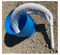
6. With a zip-tie, tie of the other end of the drainage sock around the angled end of the fill pipe
