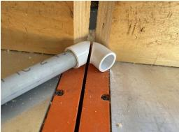
screen outside so I can see if it needs replacing. CAUTION! When cutting the elbow in half, first place it on a length of PVC to keep your hands away from the saw. Cut the elbow SLOWLY or it will shatter.
